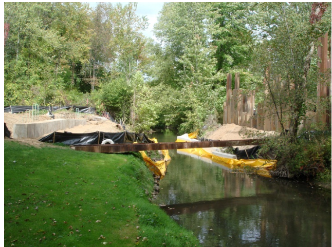
Kalamo Hwy bridge reconstruction, Eaton Twp
