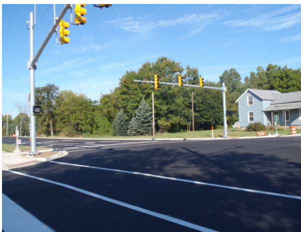
St. Joe Hwy & Broadbent Road, Delta Township
