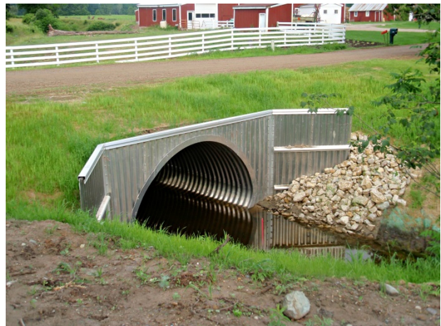
Wilson Road Culvert, Hamlin Township
