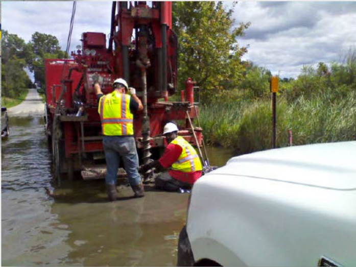
Soil Borings on Five Point Hwy, Carmel Twp
