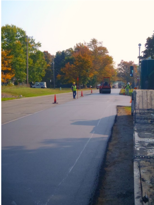
Asphalt Overlay on Packard Hwy Eaton Twp
