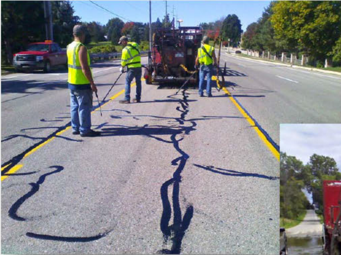
Crack Seal on Willow Hwy, Delta Twp
