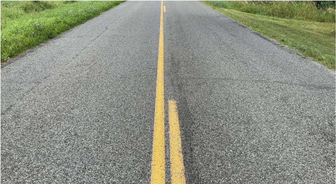
2017 Millage Project with 2024 Chip Seal
