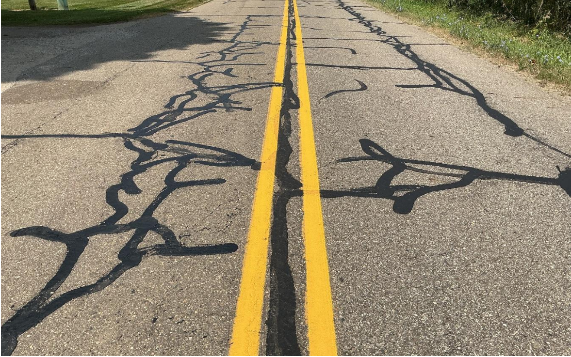
2017 Millage Project – No Surface Treatment
